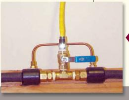
Configuration under each laboratory table consists of inlet and outlet runs of TracPipe® PS-II with vent ports connected by a copper tube jumper. This provides a continuous vent for the entire run to a suitable outdoor location. The vertical tee outlet is attached to a gas valve and then a flexible appliance connector to the table-top burner.
